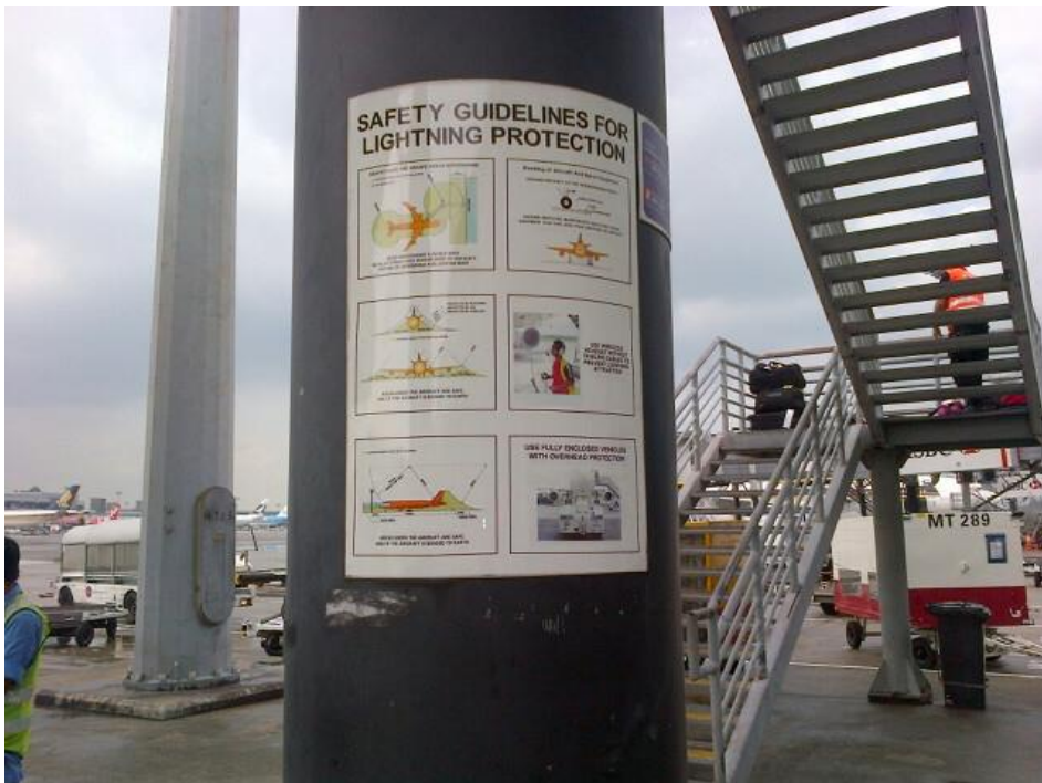
4th picture shows signs posted on all bridge columns displaying precaution needed when thunderstorm is imminent and David Clark wireless headset/system is shown as a requirement.
